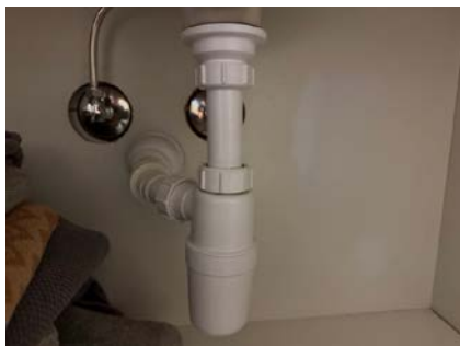
Røropplegg under servant.
