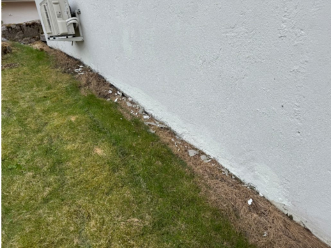
Fuktsperre delvis under terreng
