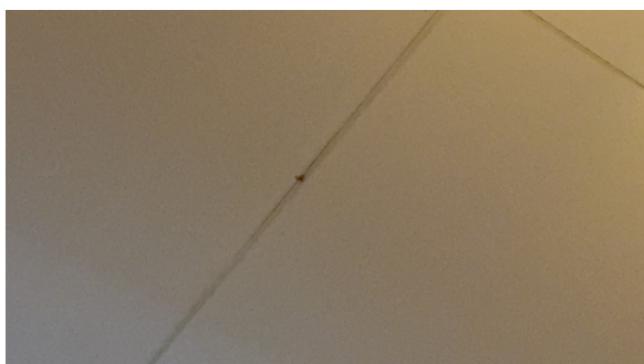
Synlig innfesting i himling.
