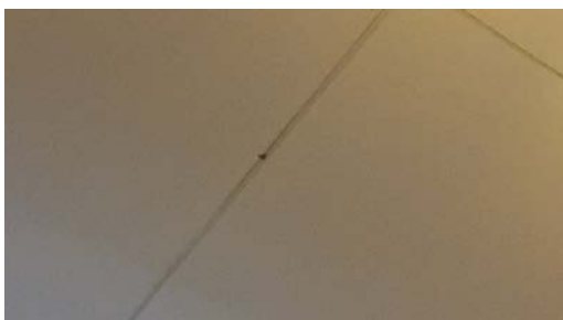
Synlig innfesting i himling.
