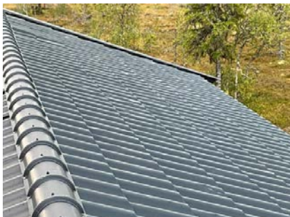
Bulker i takplater.
