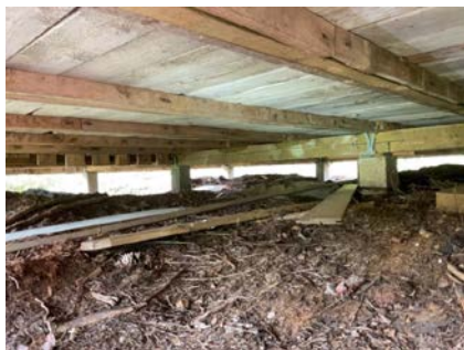
Stubbegulv under bjelkelag.
