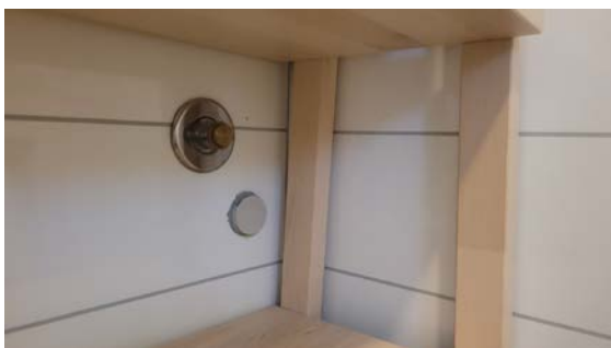
Opplegg for vaskemaskin.
