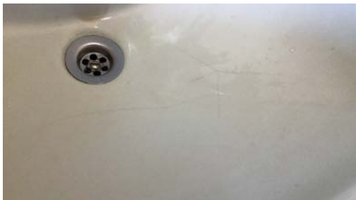
Riss i servant.
