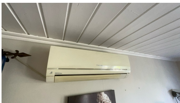
Varmepumpe innerdel.
