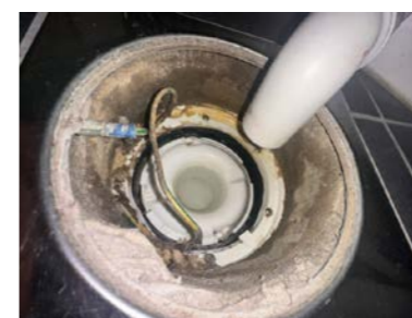
Sluk i plast, plassert under servant
