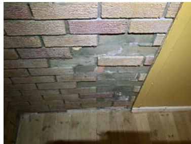
Løsnet teglforblending.
