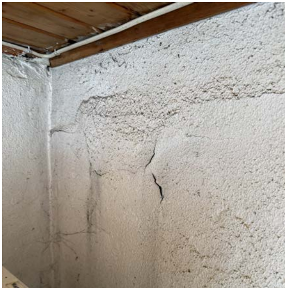
Sprekker/riss
