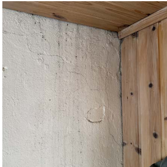
Sprekker/riss
