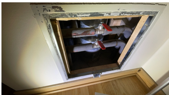
Stoppekran i luke i gang
