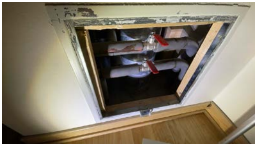
Stoppekran i luke i gang
