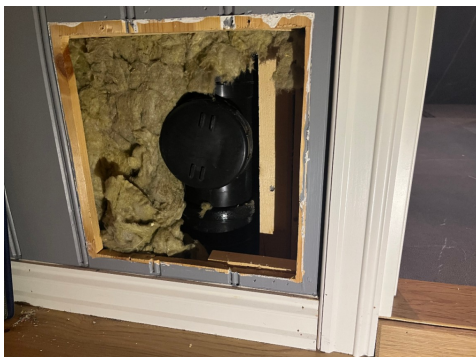
Stakeluke i vegg mot bad.
