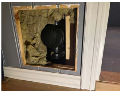
Stakeluke i vegg mot bad.
