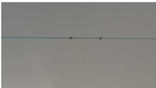
Synlig innfesting i himling.
