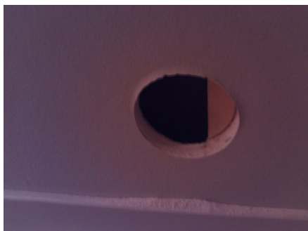
Hulltaking i utfored vegg.
