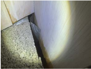
Dampsperran rundt pipen.
