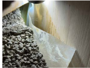
Dampsperran rundt pipen.
