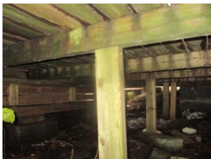
Noe enkel fundamentering.
