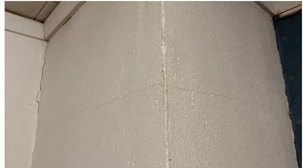
Riss i pipe
