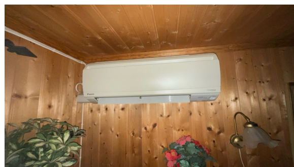
Varmepumpe innerdel.
