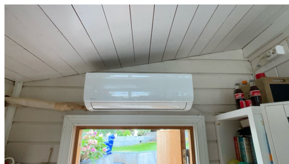
Varmepumpe innerdel.
