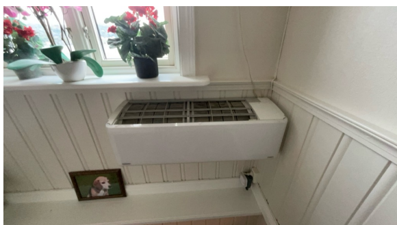
Varmepumpe innerdel.
