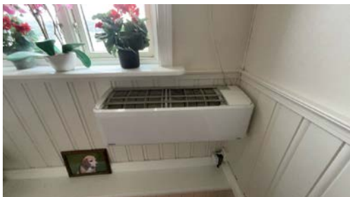
Varmpumpe innerdel.
