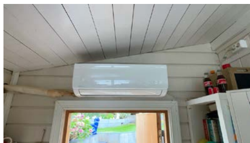
Varmepumpe innerdel.
