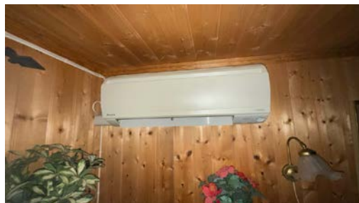
Varmepumpe innerdel.
