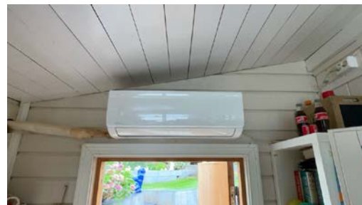
Varmepumpe innerdel.
