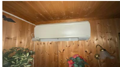
Varmepumpe innerdel.
