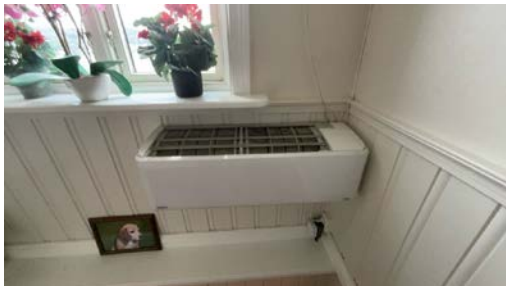
Varmepumpe innerdel.
