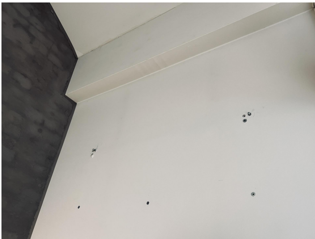
Stedvis plugg hull i veggoverflater.
