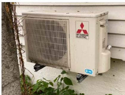
Utedel varmepumpe.
