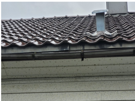
Deformert takrenne.
