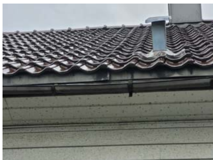
Deformert takrenne.
