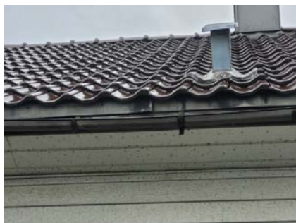
Deformert takrenne.
