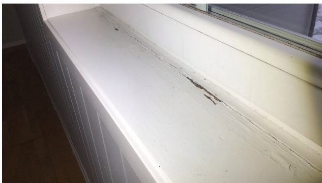
Fukt merker i foring i underkant
