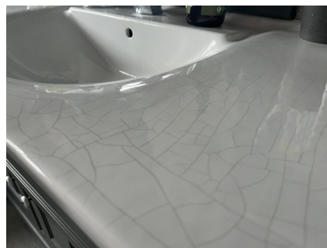
Krakelering i servant.
