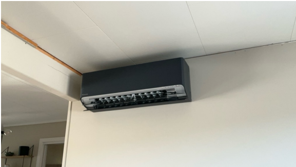
Varmepumpe innerdel.
