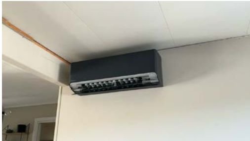
Varmepumpe innerdel.
