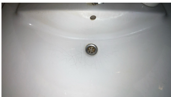
Riss i servant
