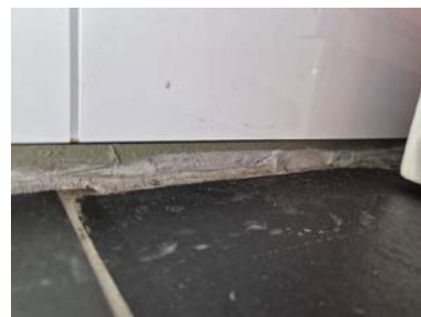
Mangler aluminiumslist.
