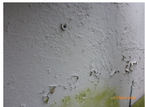
Under varmepumpe vest
