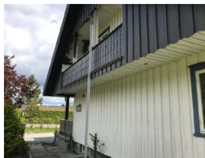
Manglende overflatebehandling.
