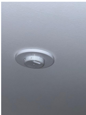
Innfelt sprinkelhode for slukking
