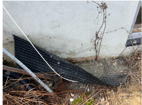
Manglende innpussing/klemplst
