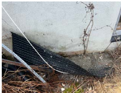
Manglende innpussing/klemmlist
