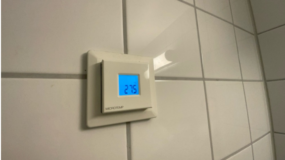
Termostatbryter for varmekabler.
