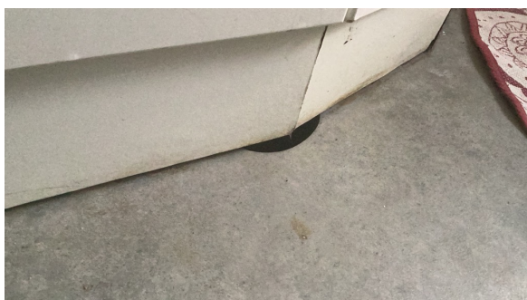
Sluk under servant.
