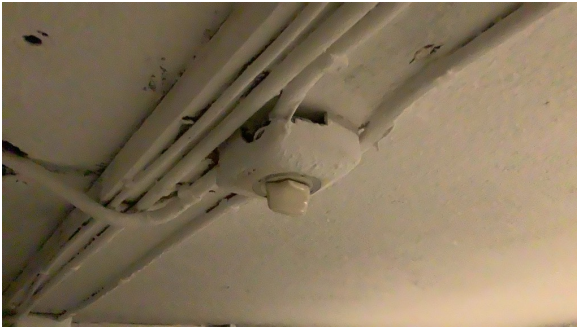
Skadet kapsling.
