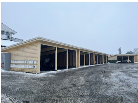
Felles carport anlegg.
