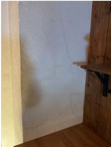
Sprekker i pipe.
