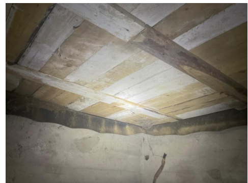
Stubbloft under trebjelkelag.
