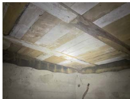
Stubbloft under trebjelkelag.
