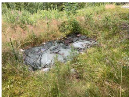
Septiktank under presenning.
