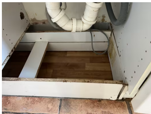
Fuktskade under vask.
